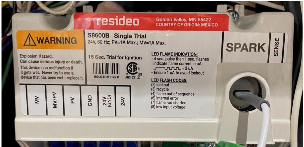
Figure 24. Intermittent ignition device front with chart of fail codes.
