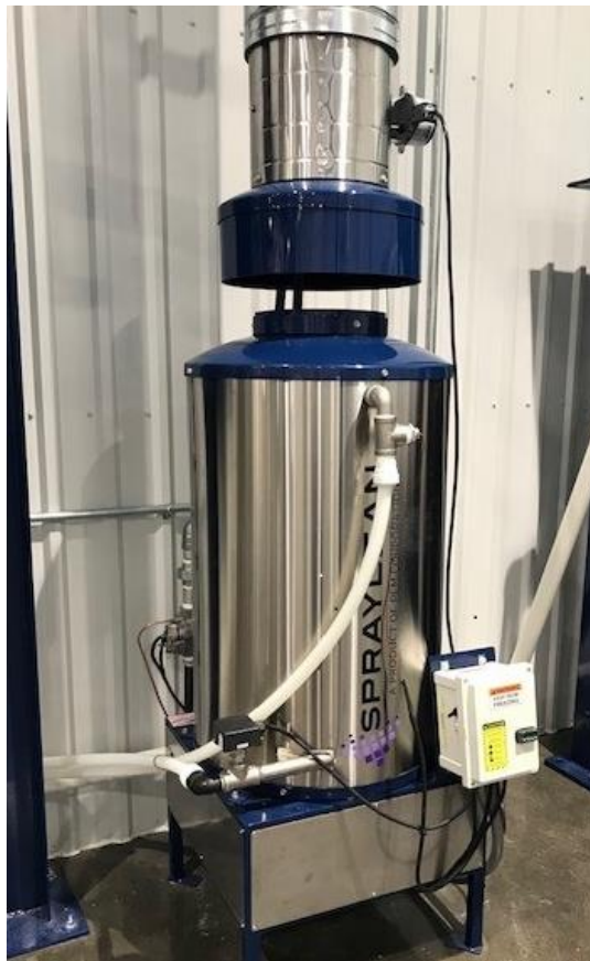
Figure 11: LP / natural gas heaters
