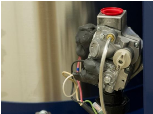
Figure 4: Gas Valve
